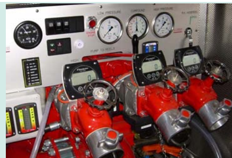
East Sussex Fire and Rescue Service Pump Bay
